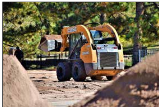
October 15: Spreading base material.
